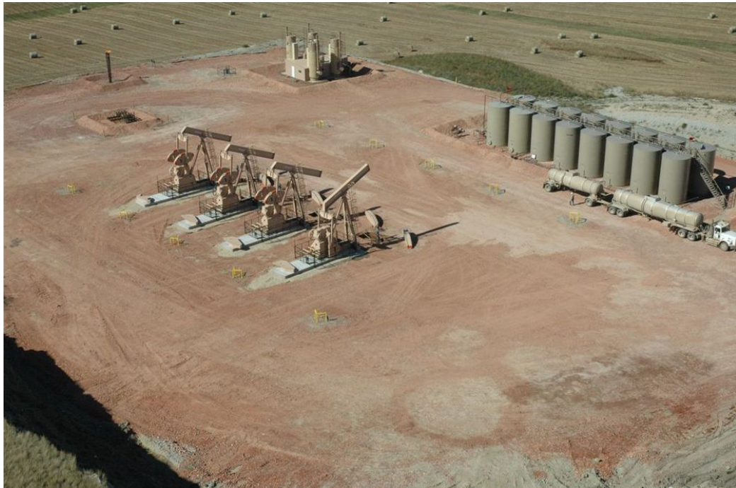
Figure 4.4: A multi-well pad site containing four wells.
